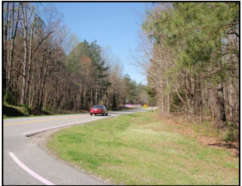
Brassfield Road looking west toward Creedmoor
