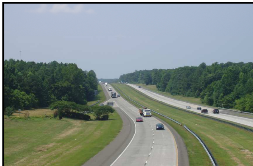
I-85 looking south from NC 96
