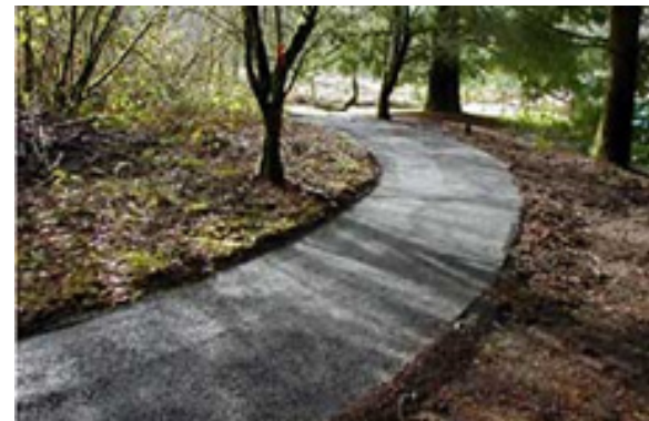
Crushed Stone Trail
