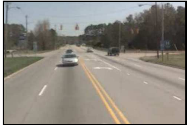
Existing Dabney Drive
