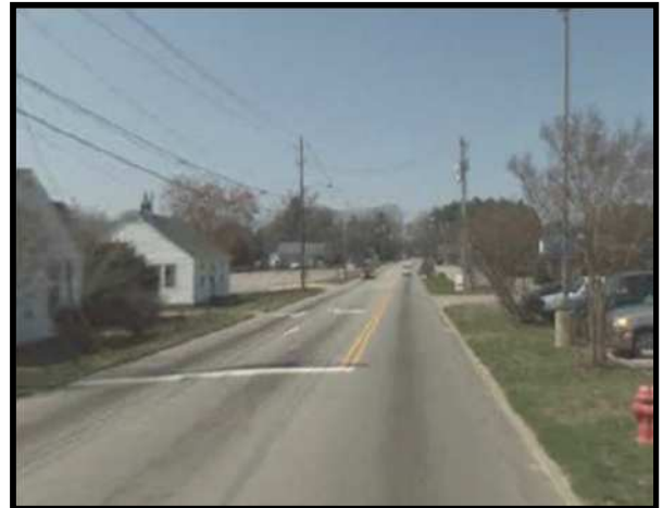
Existing Dabney Drive
